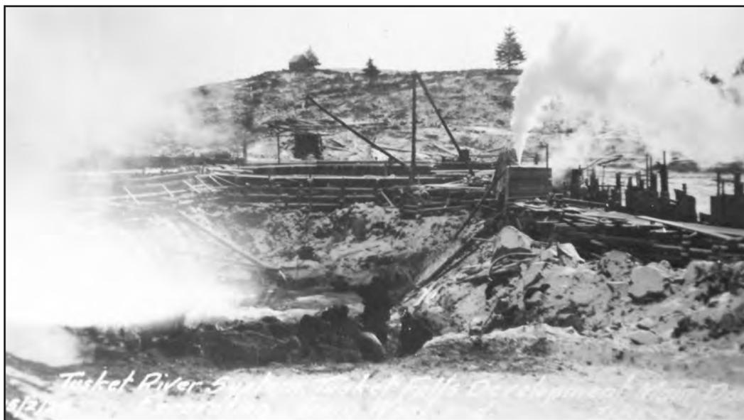
Figure 2: Excavation of the main dam in 1929 with steam powered Errie shovels (Argyle Township Court House Archives P1999-712pf).
