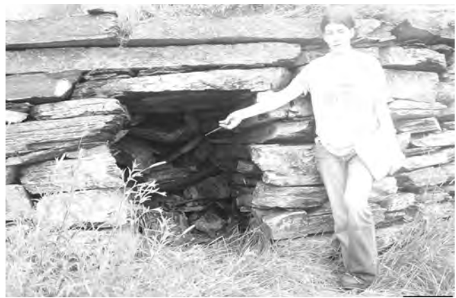
Cistern at Port Kirwan, Newfoundland (CfAf-17).
